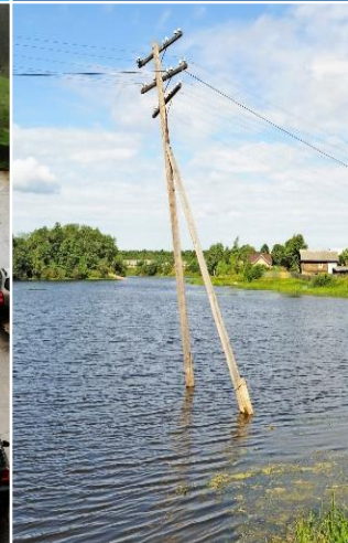
POWER AND COMMUNICATIONS
